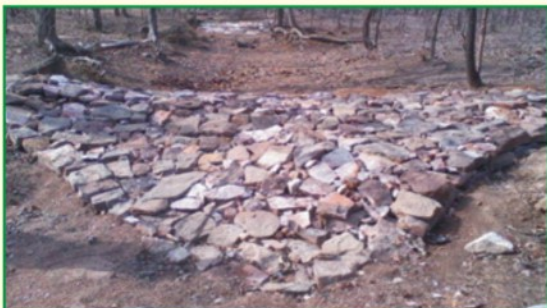
Constructed Loose Bolder Structure
